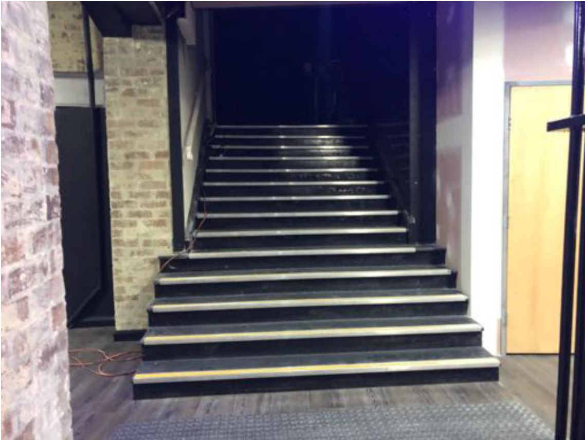
Figure 10: Stairs connecting Lot 4B to the building's common corridor
