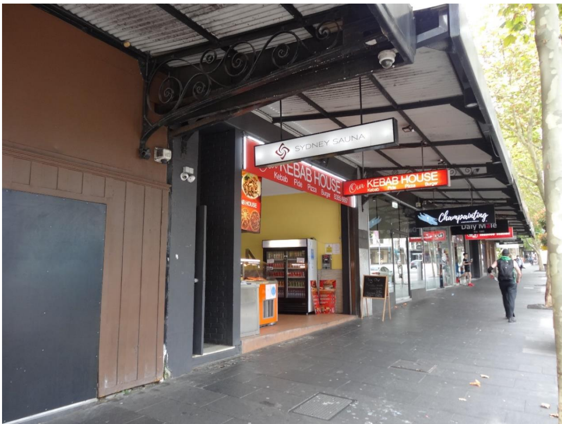
Figure 3: The site ground floor and entrance viewed from Oxford Street.
