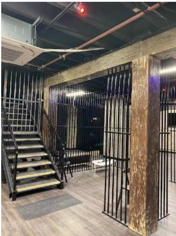
Figure 9: The stairs constructed to connect to the sex on premises above
