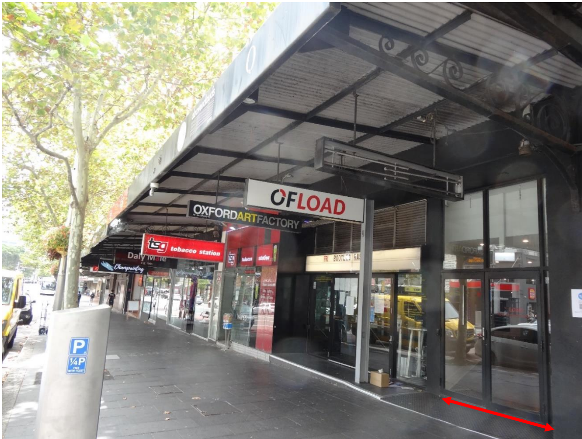
Figure 6: The entrance to the common corridor and lift access
