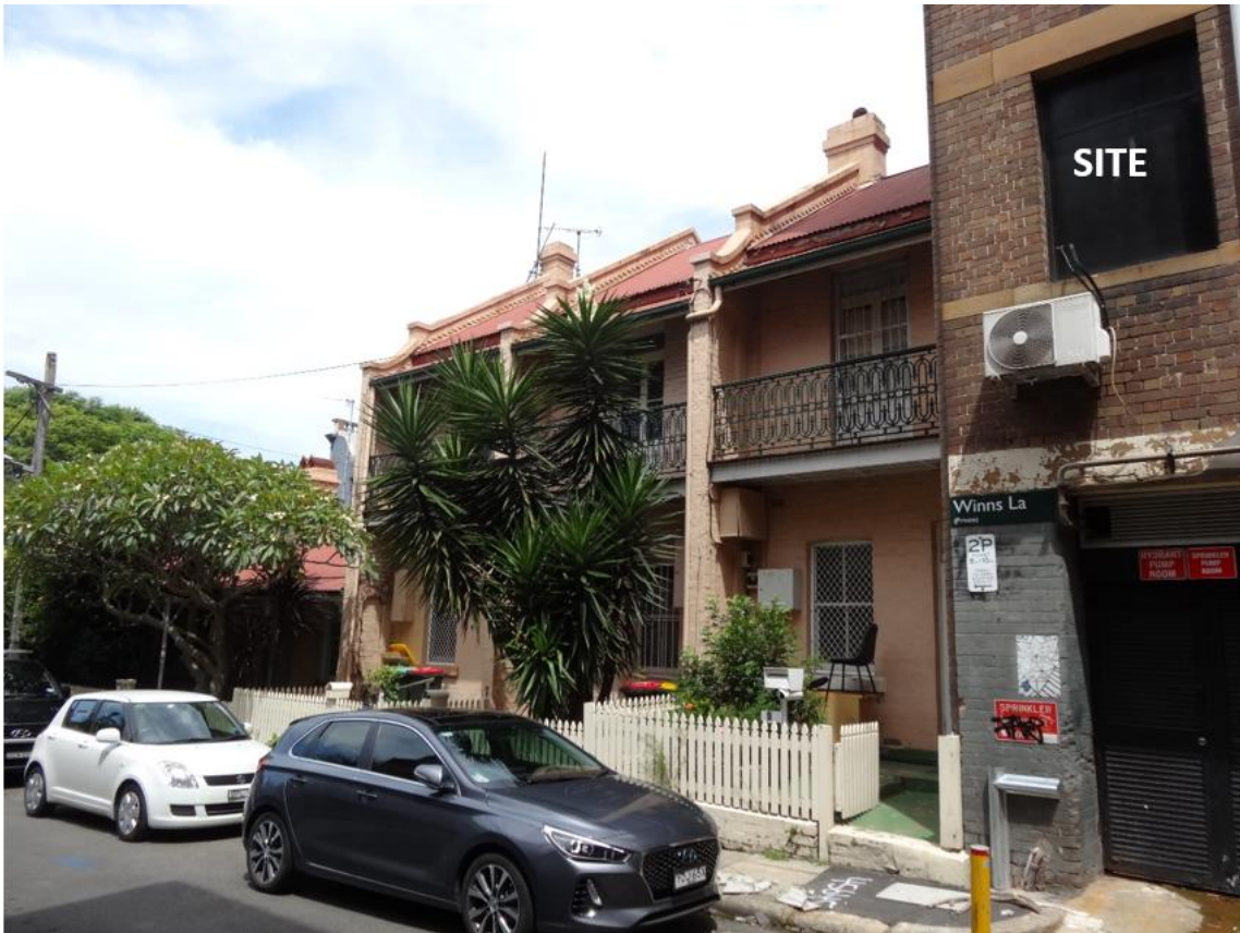
Figure 18: Residential terraces at 5-17 Norman Street
