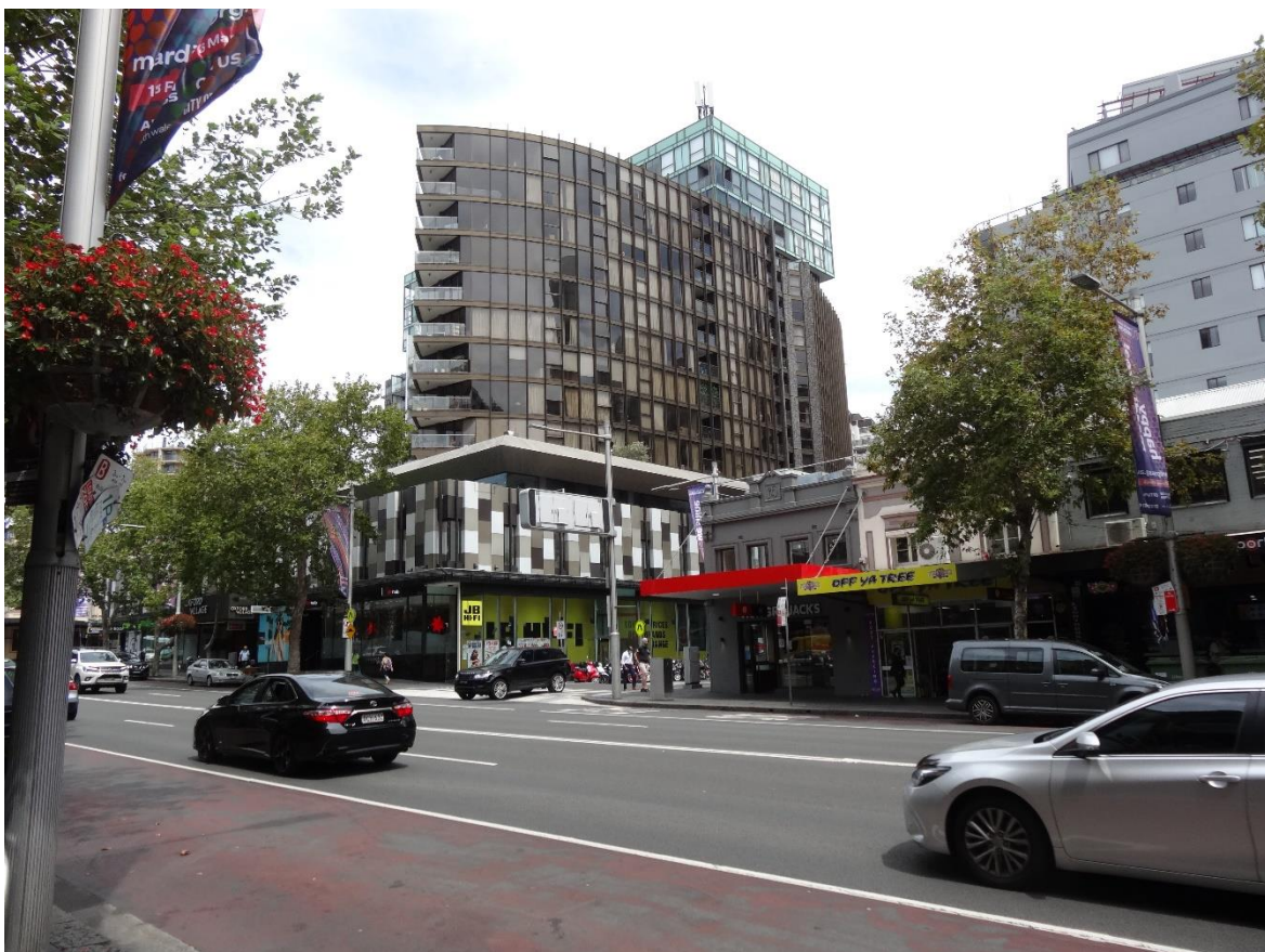
Figure 19: Mixed use development on the opposite side of Oxford Street (number 55-73)
